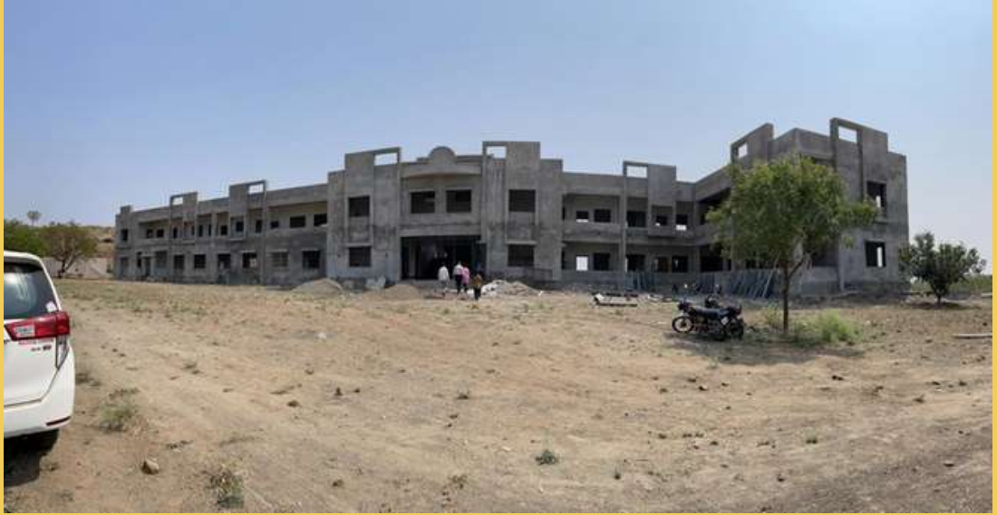
Current Status of the Construction
